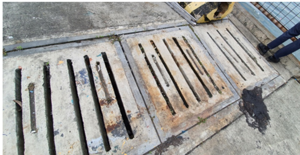
Figure 49. Drainage Outfall in Manila North Harbor last October 20, 2021
