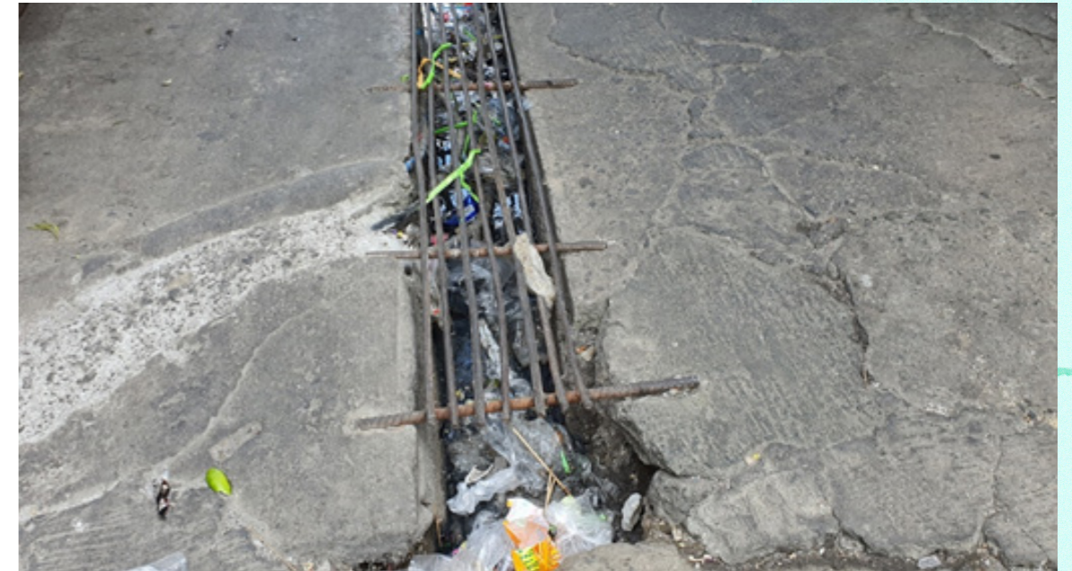
Figure 50. Storm Drain in Barangay 20 last October 20, 2021
