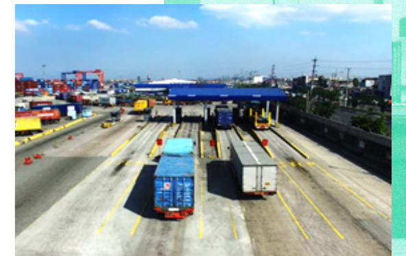
g. Weigh Bridge Area
