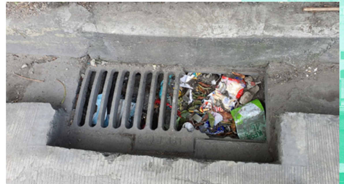
Figure 51. Storm Drain in Barangay 275 last October 21, 2021
