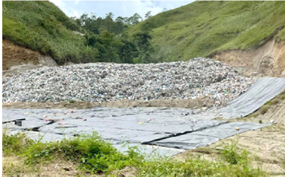
Figure 17. EcoWaste Treatment and Disposal Facility last October 14, 2021
