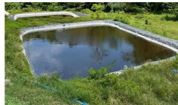
Figure 18. Leachate Ponds at the City SLF last October 14, 2021
